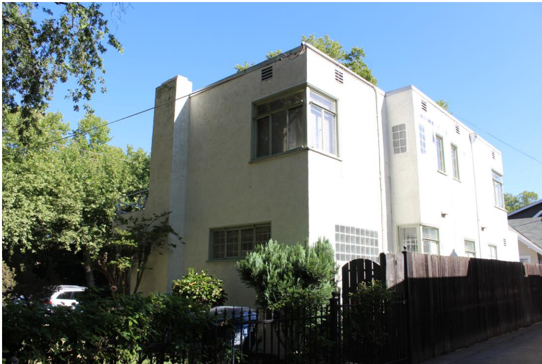
Photograph 3: 2131 17 th Street, south and east elevations, camera facing northwest, June 15, 2021.
