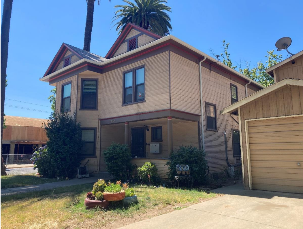
Photograph 4: 1830 T Street, north and west elevations, camera facing southeast, June 15, 2021.
