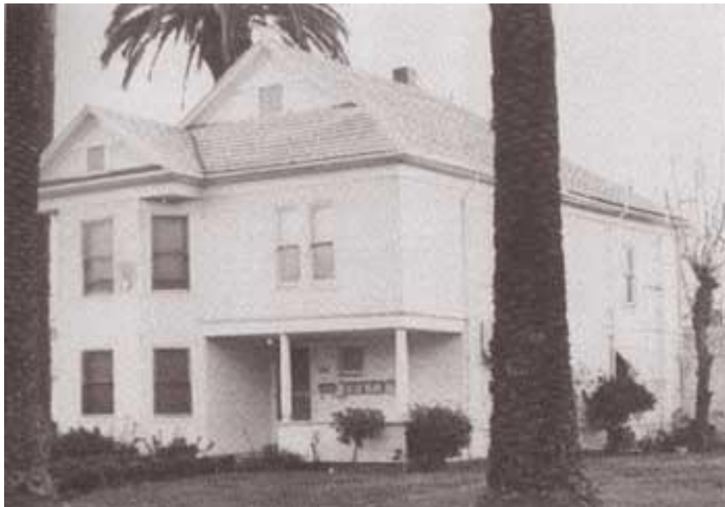
Figure 2: 1830 T Street, north and west elevations, 1942.
