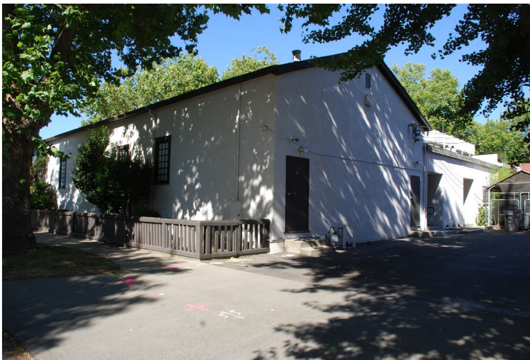
Photograph 4: Northwest and southwest elevations, camera facing northeast, June 15, 2021.
