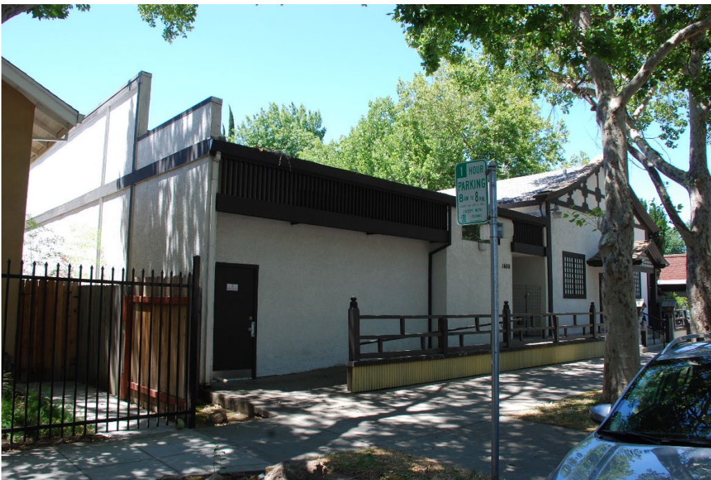
Photograph 3: 1404 and 1400 U Street, southeast and northeast elevations, camera facing southwest, June 15, 2021.
