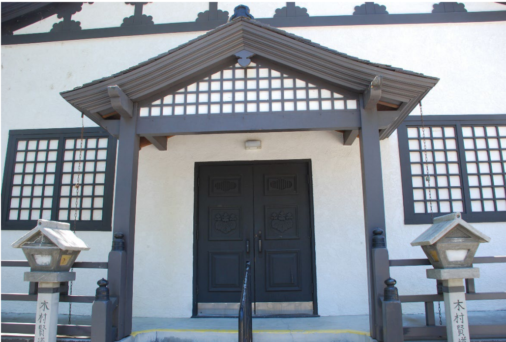
Photograph 2: Detail, main entrance, main (northeast) elevation, June 15, 2021.
