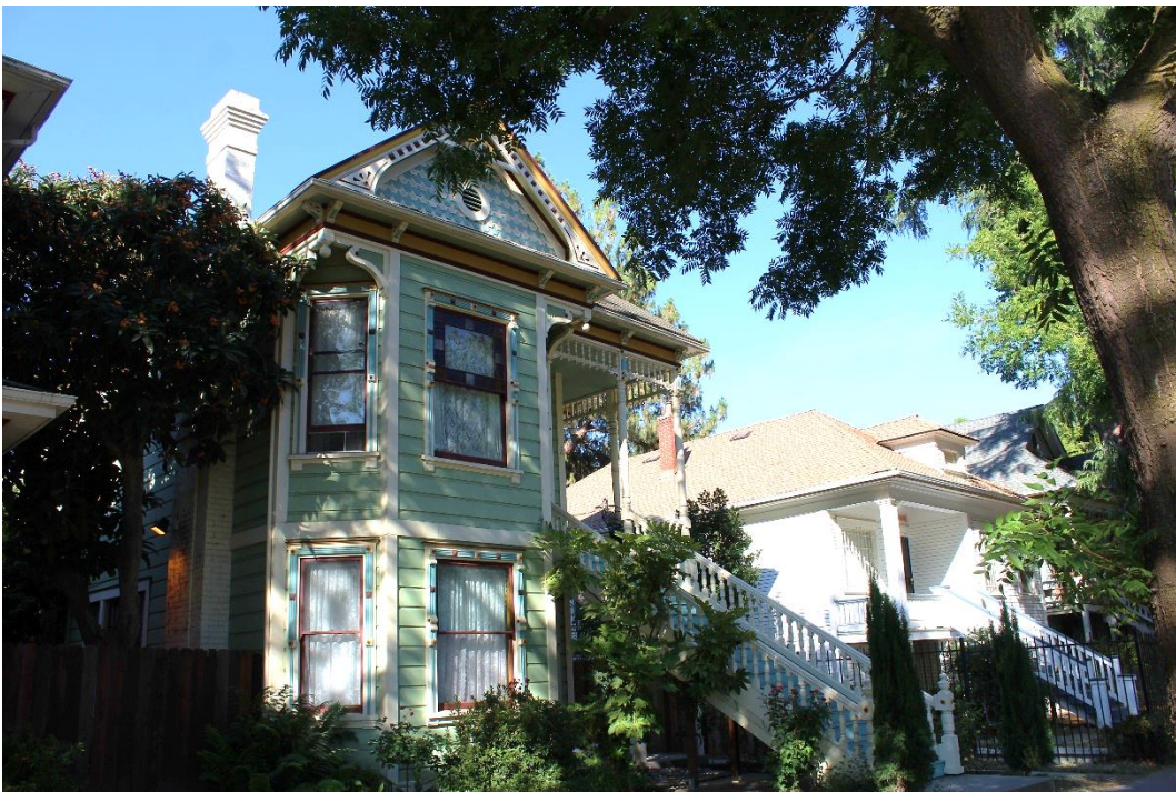
Photograph 4: 1722 S Street, northeast elevation, camera facing southwest, June 15, 2021.
