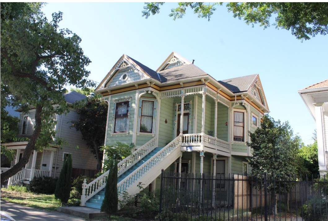
Photograph 3: 1722 S Street, northeast and northwest elevations, camera facing south, June 15, 2021.
