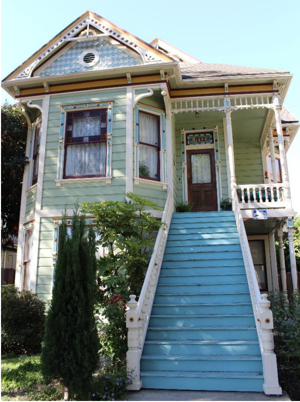
Photograph 2: 1722 S Street, northeast elevation, camera facing southwest, June 15, 2021.
