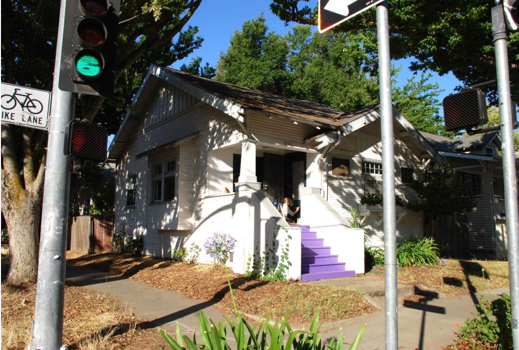
Photograph 2: 1830 V Street, east and north elevations, camera facing southwest, June 15, 2021.
