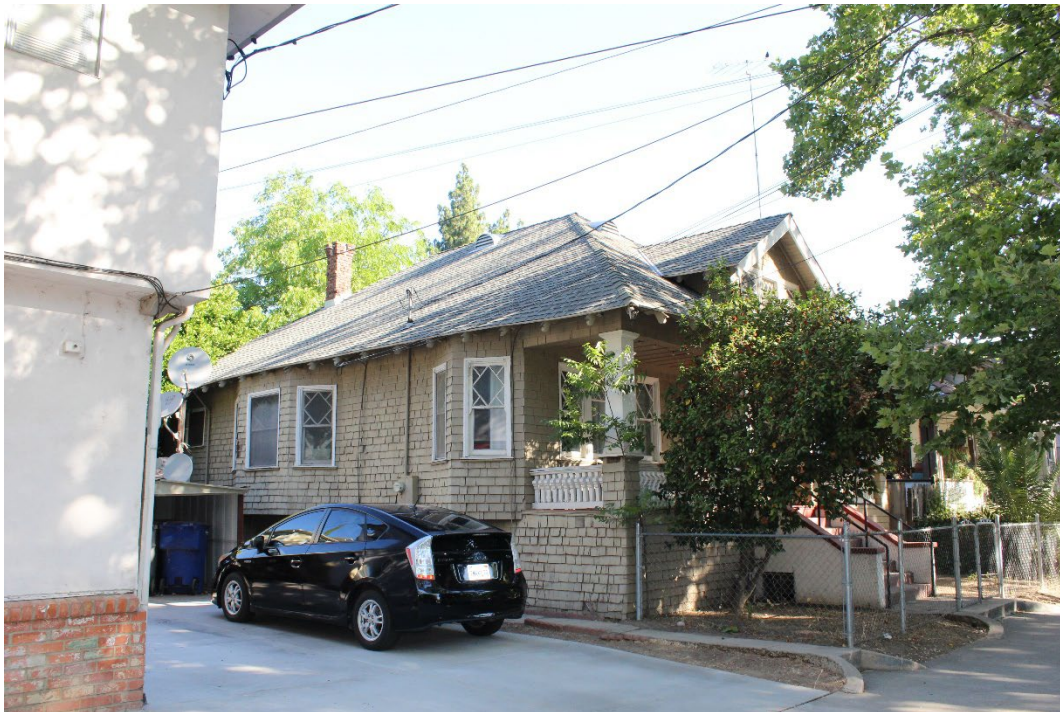
Photograph 2: 1920 18 th Street, east elevation, camera facing northwest, June 15, 2021.
