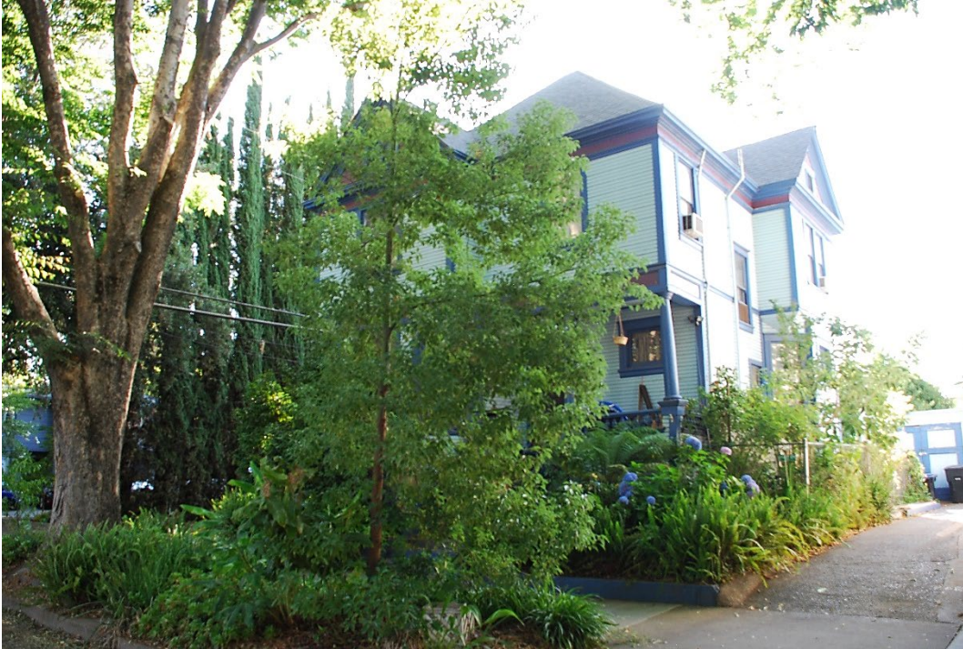
Photograph 2: 2117 18 th Street, west and south elevations, camera facing northeast, June 15, 2021.
