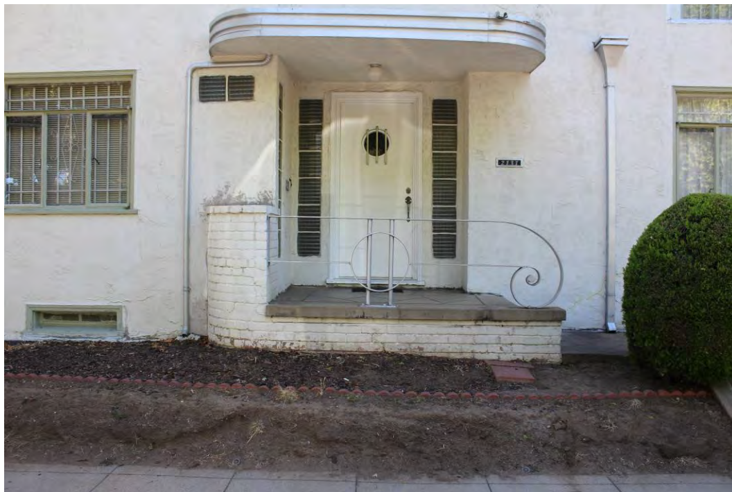
Photograph 4: 2131 17 th Street entrance, west elevation, camera facing east, June 15, 2021.
