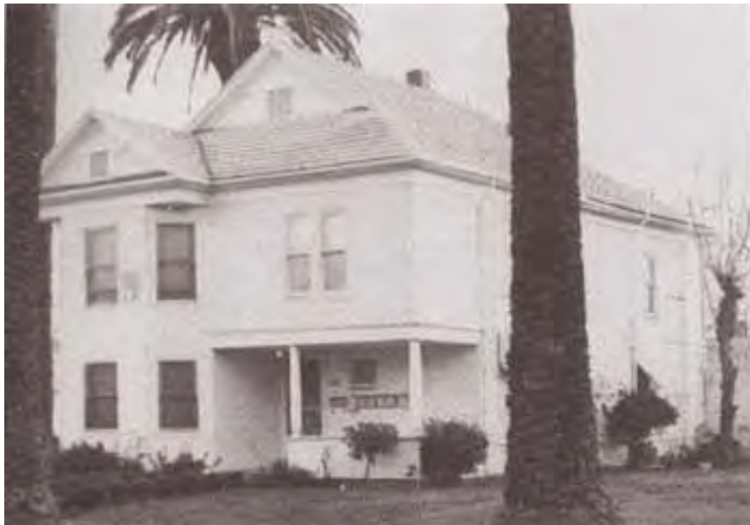
Figure 2: 1830 T Street, north and west elevations, 1942.
