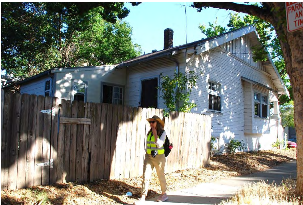
Photograph 3: 1830 V Street, south and east elevations, camera facing northwest, June 15, 2021.
