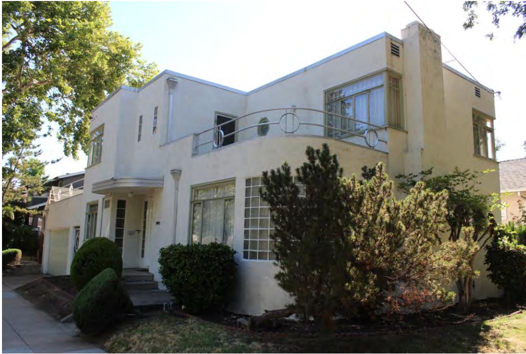
Photograph 1: 2131 17 th Street, west and south elevations, camera facing northeast, June 15, 2021.
