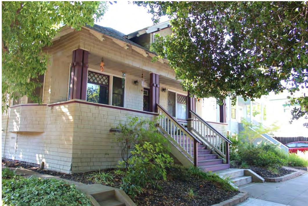
Photograph 2: 1917 17 th Street, north and west elevations, camera facing southeast, June 15, 2021.
