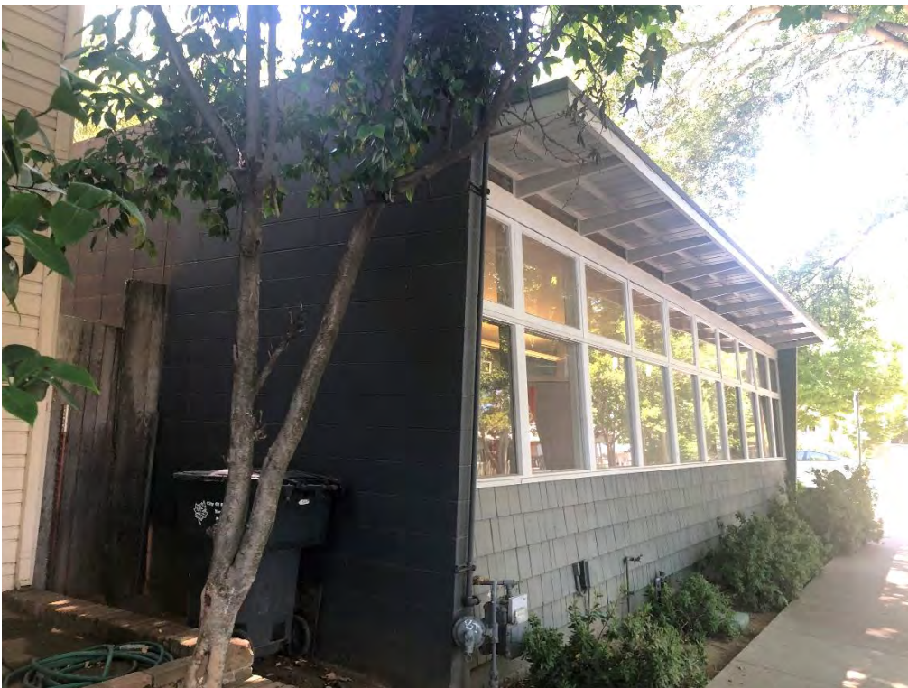
Photograph 3: 2203 13 th Street, east and north elevations, camera facing southeast, June 15, 2021.
