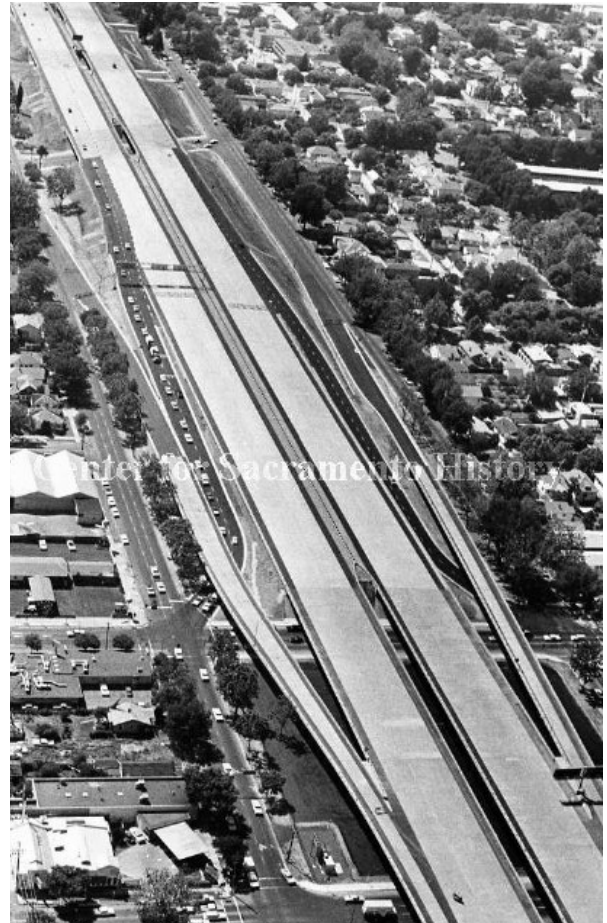
Figure 29: Golden State Highway, view from 17 th Street, 1967 (Center for Sacramento History).
