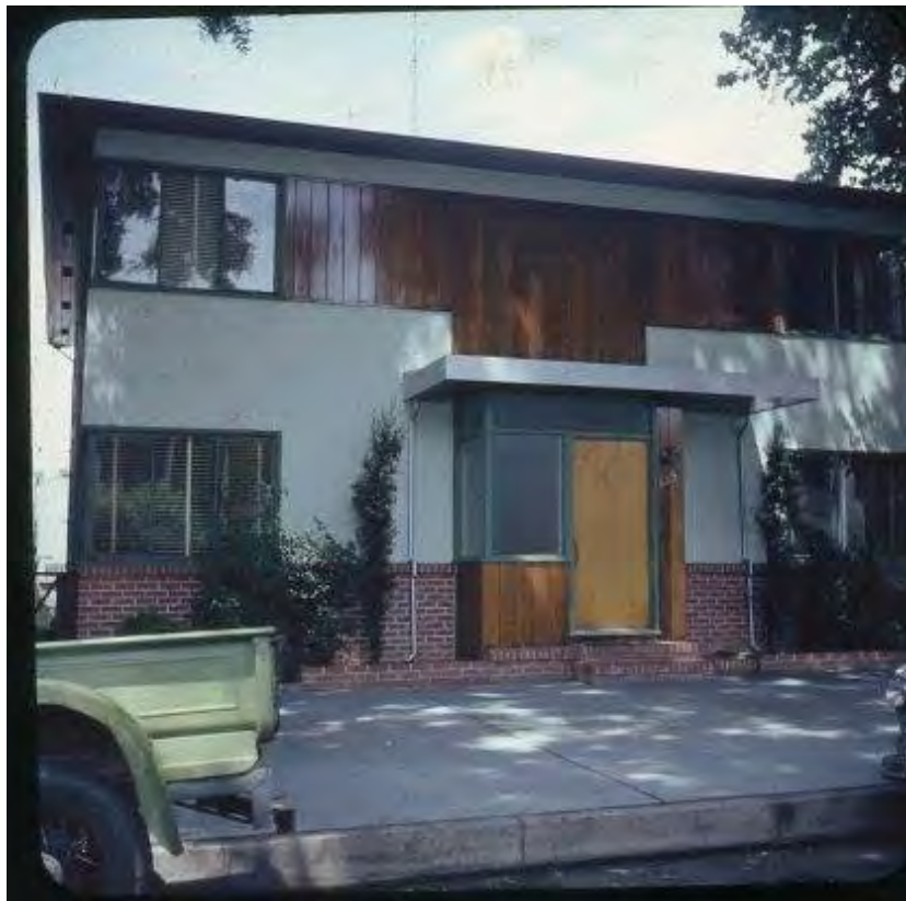
Figure 40: Apartment building at 615 O Street prior to move, Sacramento Business and Taxpayers Association, 1954 (Collection of William Burg).
