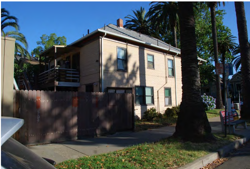
Photograph 3: 1830 T Street, south and east elevations, camera facing northwest, June 15, 2021.
