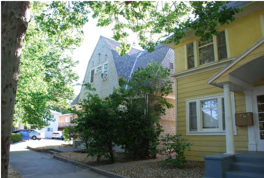
Photograph 2: 2017 18 th Street, west and south elevations, camera facing northeast, June 15, 2021.
