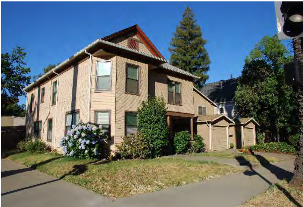
Photograph 1: 1830 T Street, east and north elevations, camera facing southwest, June 15, 2021.
