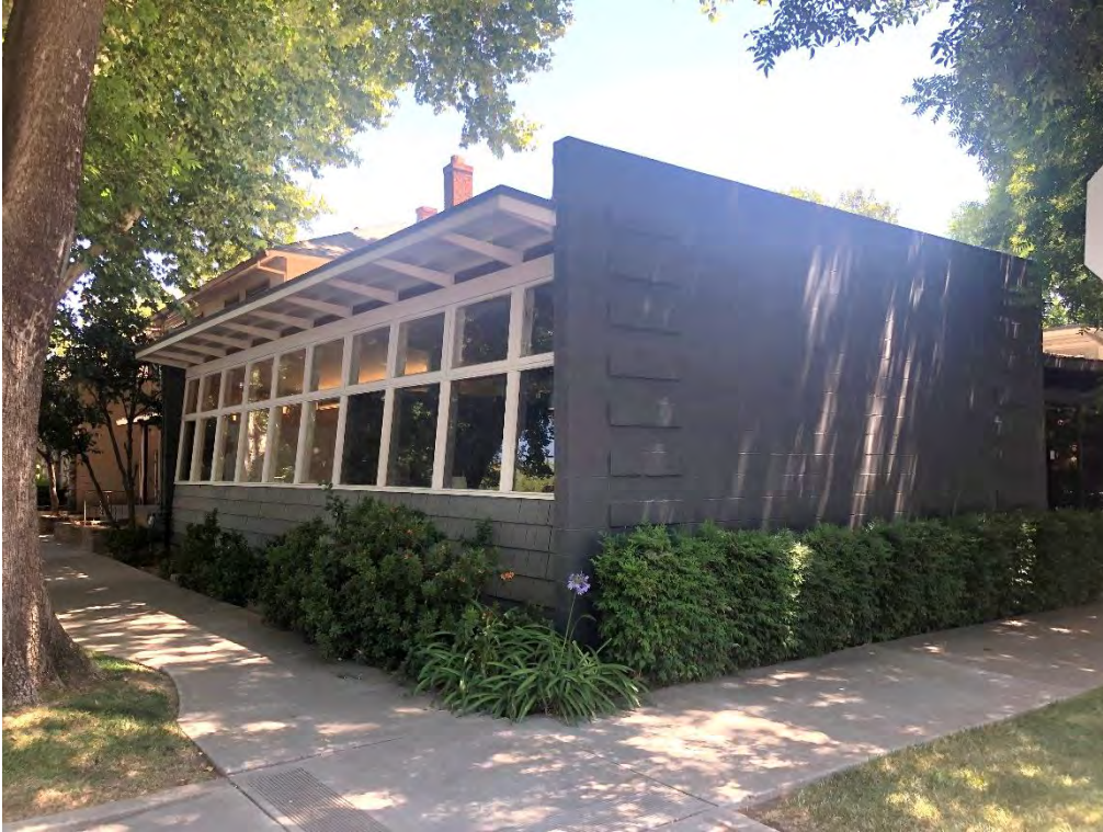
Photograph 2: 2203 13 th Street, north and west elevations, camera facing southeast, June 15, 2021.
