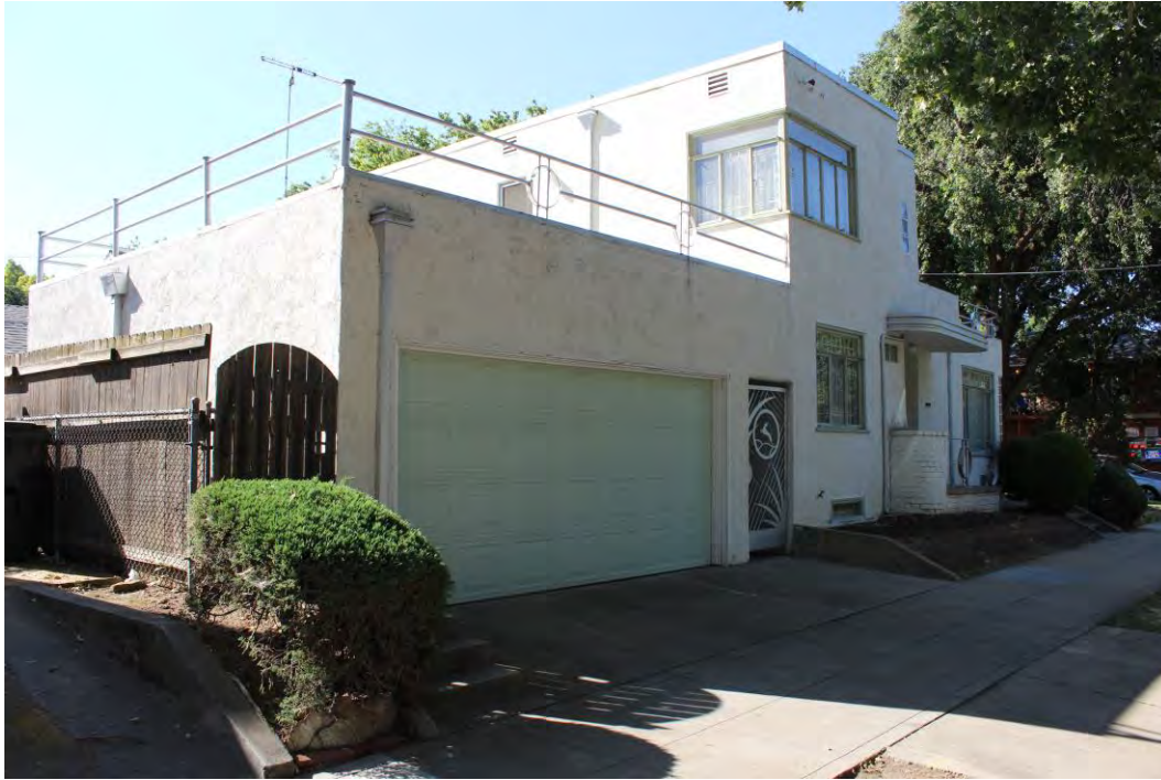
Photograph 2: 2131 17 th Street, north and west elevations, camera facing southeast, June 15, 2021.
