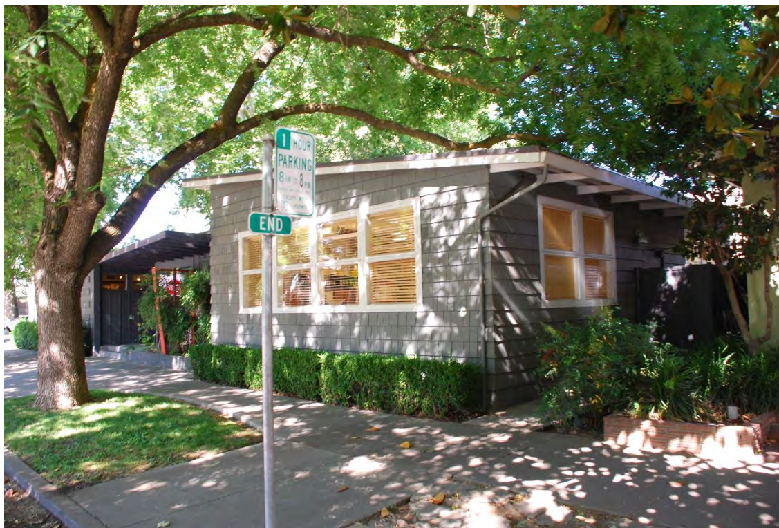
Photograph 4: 2203 13 th Street, west and south elevations, camera facing northeast, June 15, 2021.
