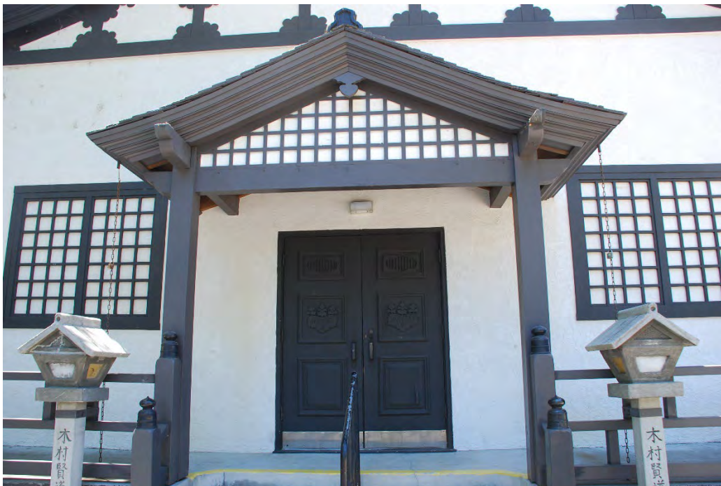
Photograph 2: Detail, main entrance, main (northeast) elevation, June 15, 2021.
