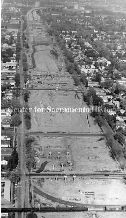
Figure 28: Demolished area of Richmond Grove during freeway construction, view from 19 th Street, 1966 (Center for Sacramento History).
